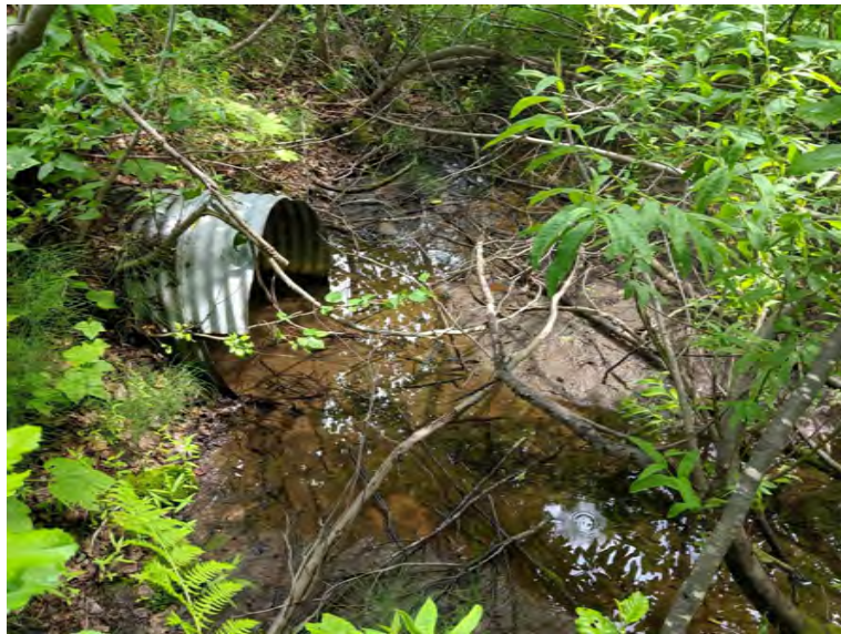
Existing Culvert Inlet
