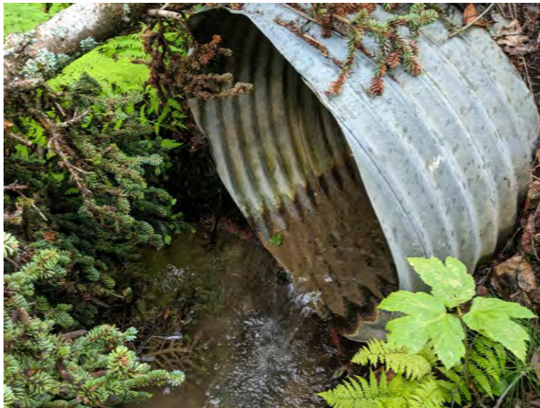
Existing Culvert Outlet
