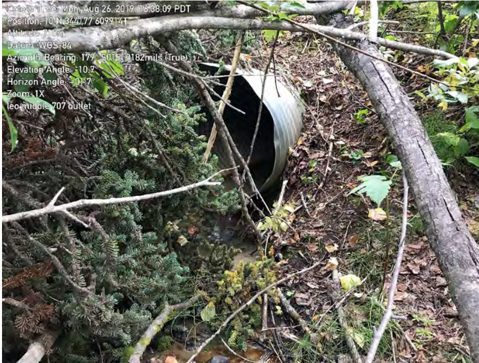
Photo 2. Photo of the culvert outlet.
