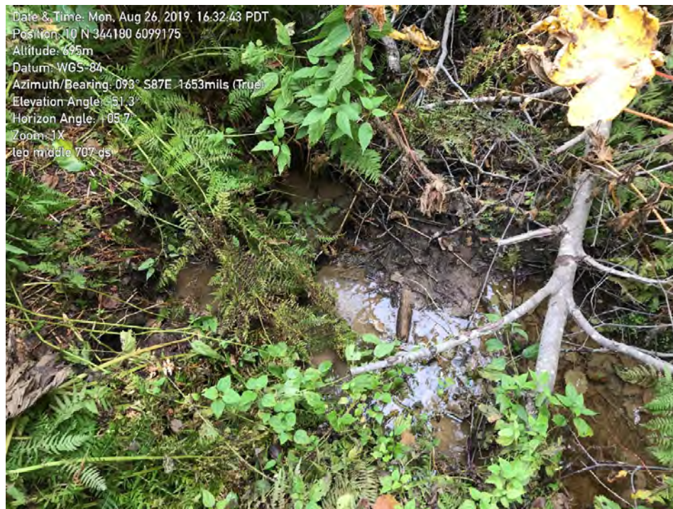
Photo 4. Photo looking across the small channel, downstream of the culvert.
