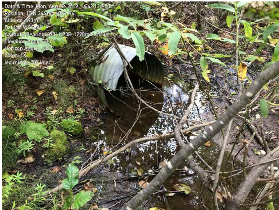
Photo 3. Photo of the culvert inlet.
